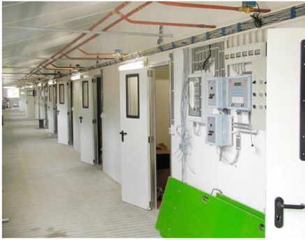
CORRIDOR WITH INTERIOR DOORS AND WINDOWS
